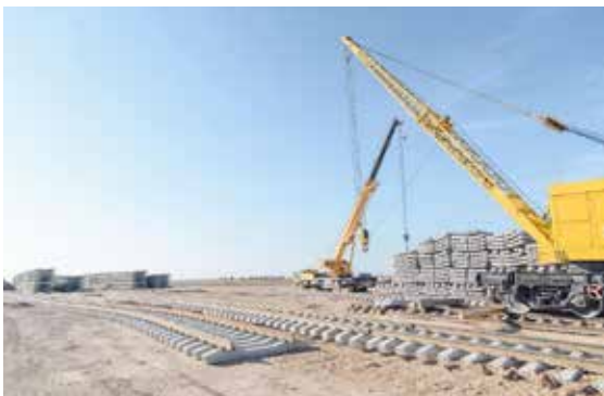
Figure 3e: Ground imagery of a DMR construction site featuring the large yellow crane, stacks of concrete rail ties, and freshly laid track to facilitate supply transport. Source: KTZ official Telegram Channel.
