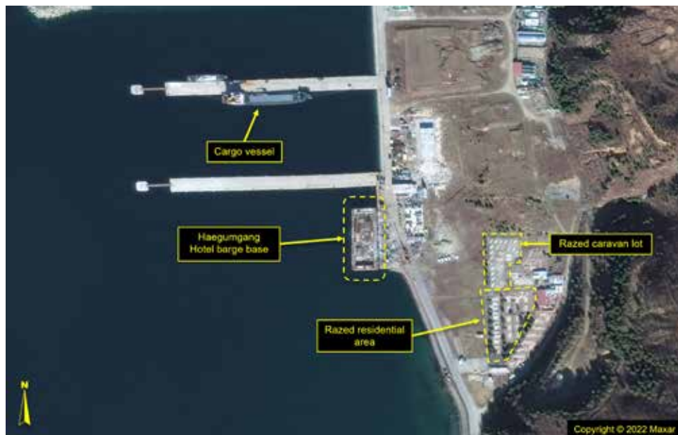
Figure 3. Imagery from December 2022 shows caravan and residential areas have been razed. Debris is observed on the foundation of the Haegumgang Hotel, but the structure no longer is in the port.
