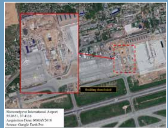
Sheremetyevo International Airport, Western Military District: Between 2078 and 2020, the airport demolished a previously standing terminal building and replaced it with a new terminal section.
