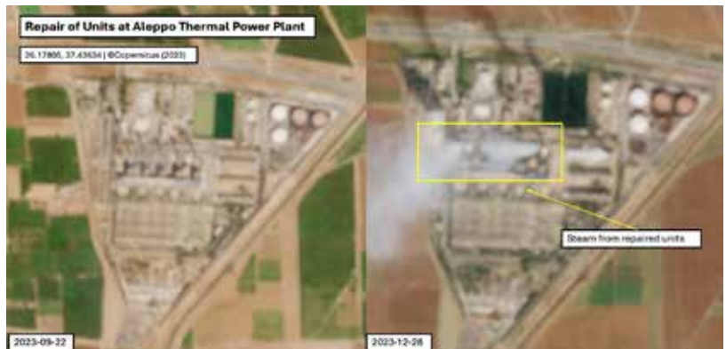
Figure 3: Sentinel imagery showing the restoration of units at the Aleppo Thermal Power Plant.
