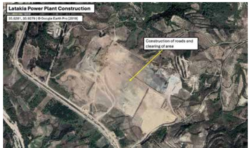
Figure 1: Annotated imagery of the preparations for construction of the Latakia Power Plant.
