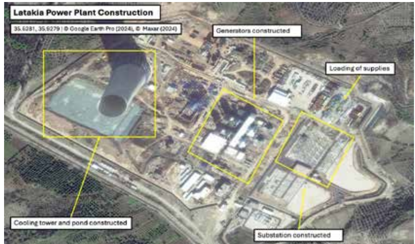
Figure 2: Annotated imagery of the progress made on Latakia Power Plant over five years.
